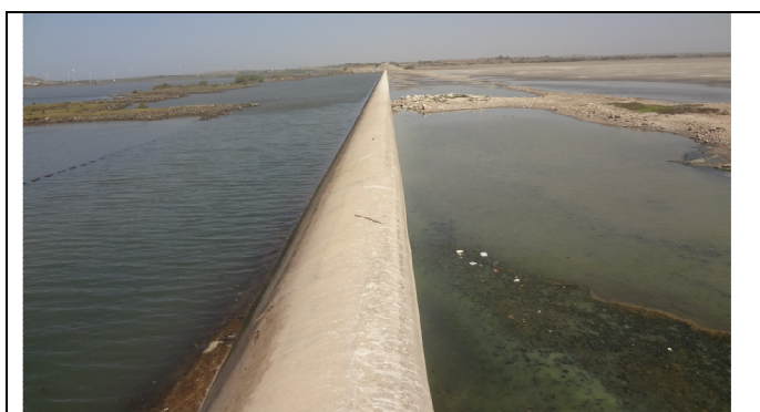
Plate No. 5.3 Field Photograph Showing Waste Weir of Medh Creek TR
