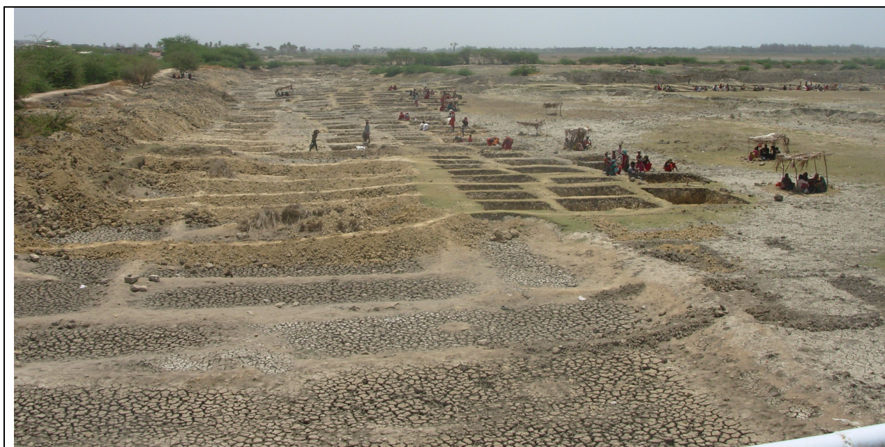
Plate No. 4.1 Desilting Activities in VasoJ Tidal Regulator
